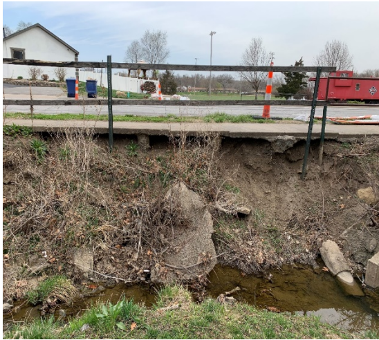
Along Main Street – Bank erosion under sidewalk
