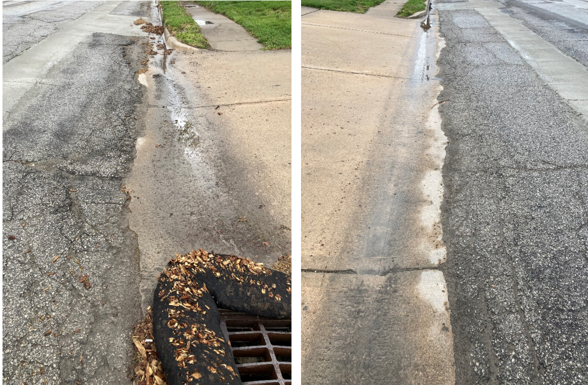
Irregular gutter along South side of Main St
